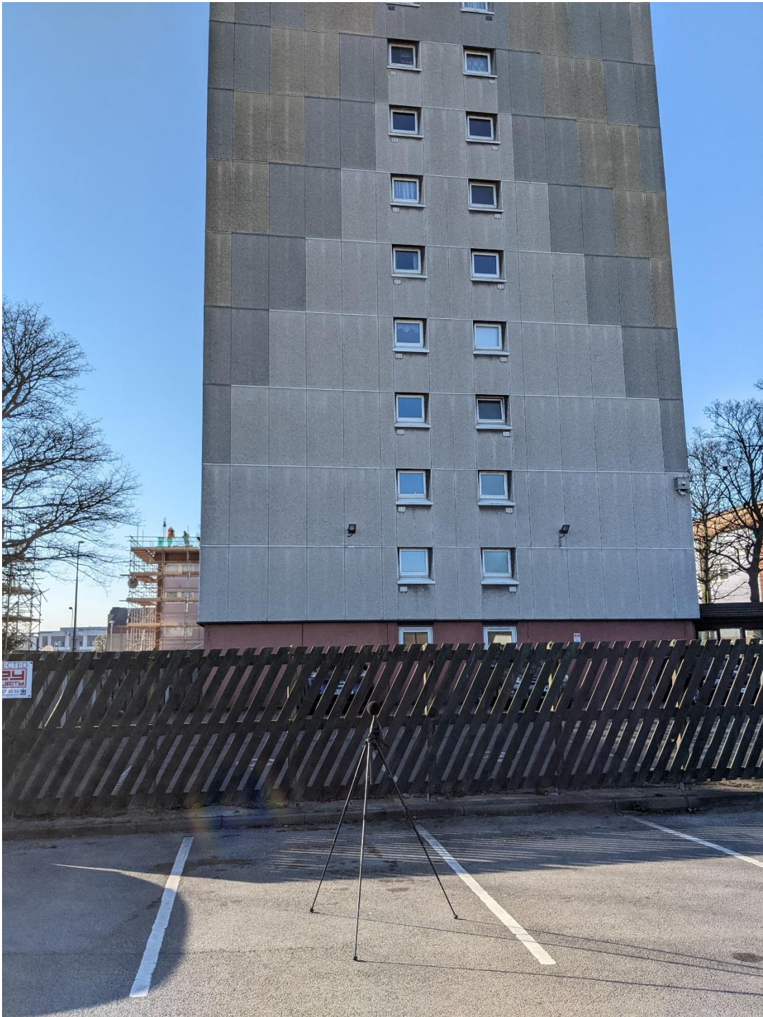
Figure 29: R11 King's Court Noise Monitoring Setup
